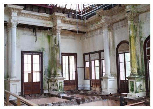
• Critical roof leaks throughout the building and ad hoc temporary solutions to stem the ingress of rain water or minimize the negative effects.
